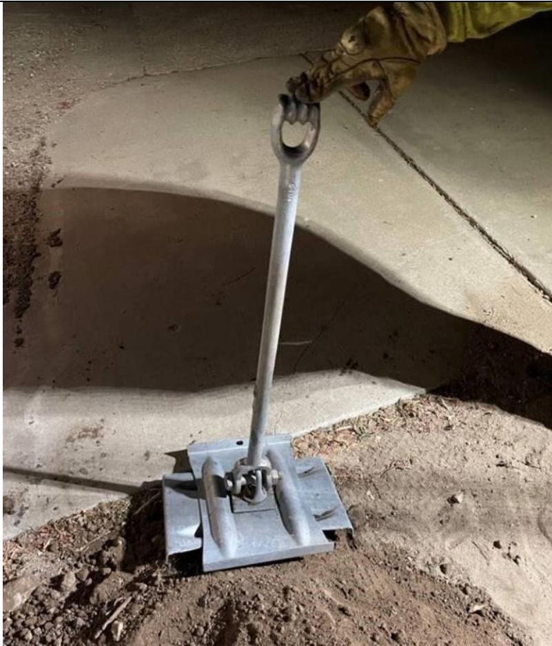
2' extension rod connected directly to a plate anchor utilizing an I-bolt
