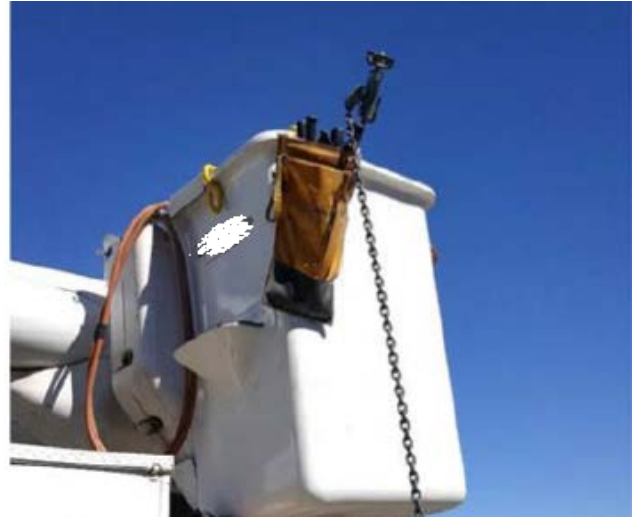
Figure 1. Example of how the pole band was placed
